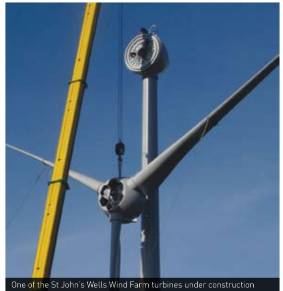
One of the St John's Wells Wind Farm turbines under construction
